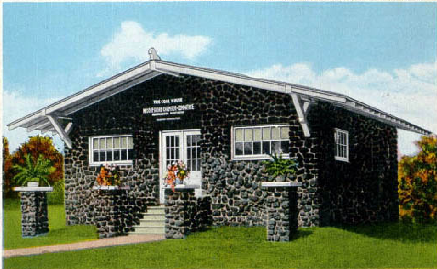
Built Entirely of Kentucky Coal
